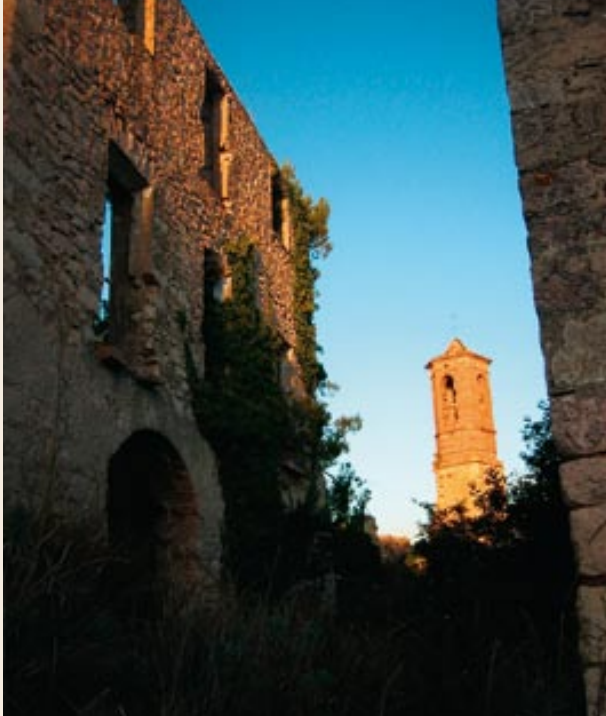
Derelict houses and streets of Selma
