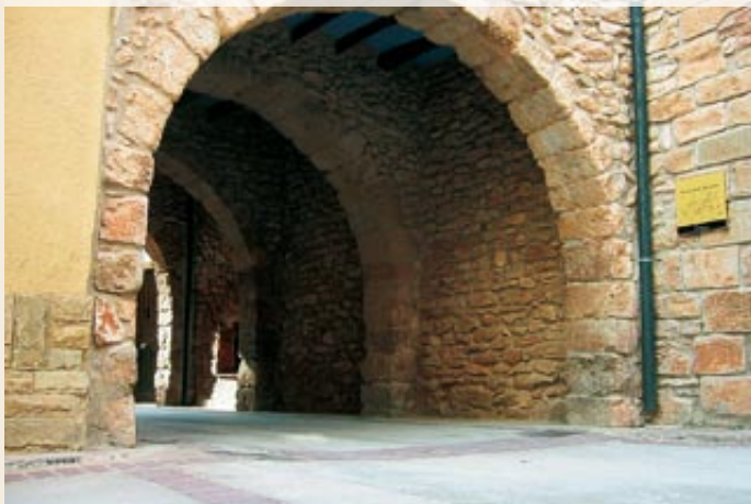
Portal on Carrer Trinitat del Pla, close to the Ajuntament
